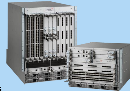
Ethernet Fabrics Data Center Access/Aggregation
