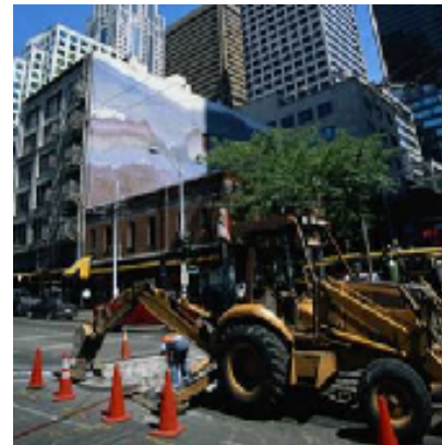
Cut cables and power
