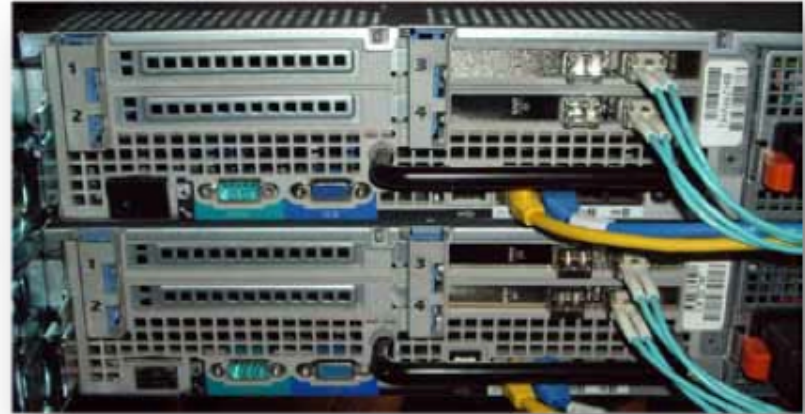
10GbE Server Connections
